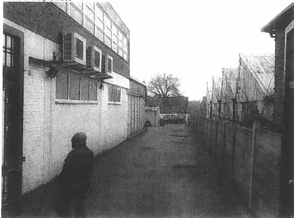
Photo of the premises
